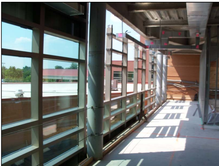
Figure 13, left – Interior view of west elevation curtain wall system under construction. Personal photograph taken by Chris Pozza.
